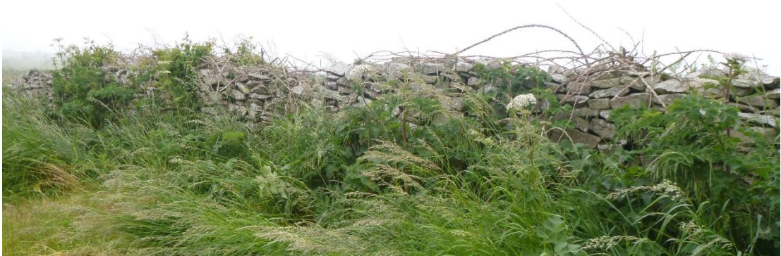
Photo 18. Illustrative image of dry stone walls separating fields.
