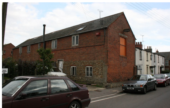
Figure 108: Warehouse, 80 North Allington.
