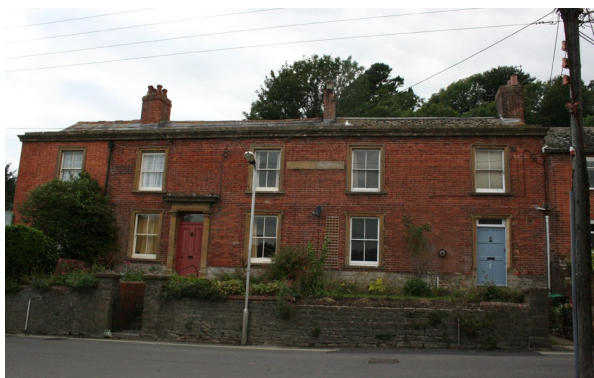
Figure 111: Former Hospital, 67-69 North Allington.
