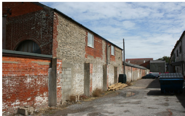
Figure 57: Former twine store and covered walk behind No. 40 St Michael's Lane.
