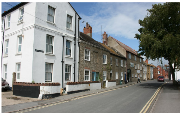
Figure 53: View north along St Michael's Lane.
