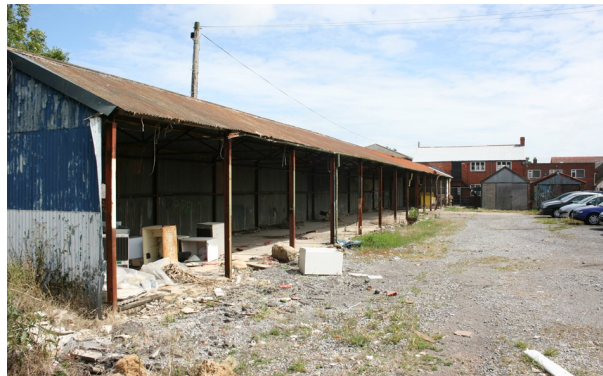
Figure 58: Corrugated iron covered ropewalk, St Michael's Lane.
