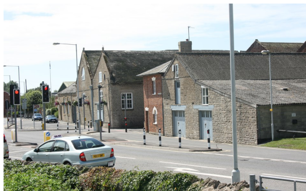
Figure 191: Old Brewery with Mineral Water Factory and brick Toll House in foreground.
