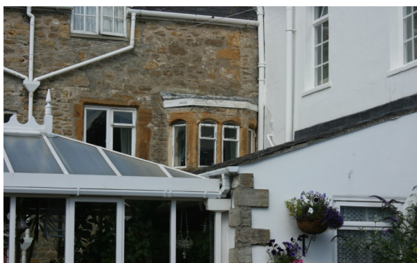
Figure 15: Oriel window said to be part of prior's house, Hospital of St John the Baptist, rear of 124-8 East Street.
