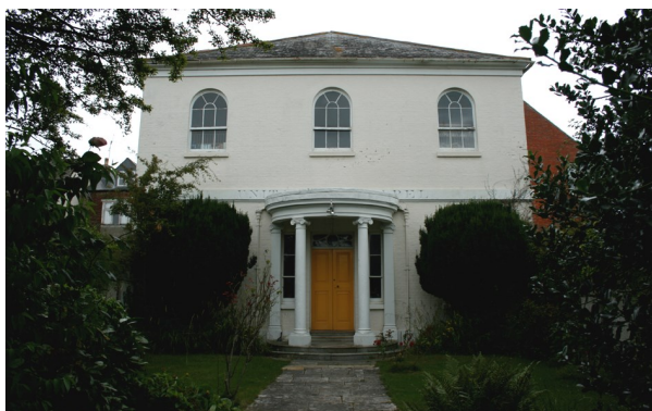
Figure 20: Unitarian Chapel, East Street.
