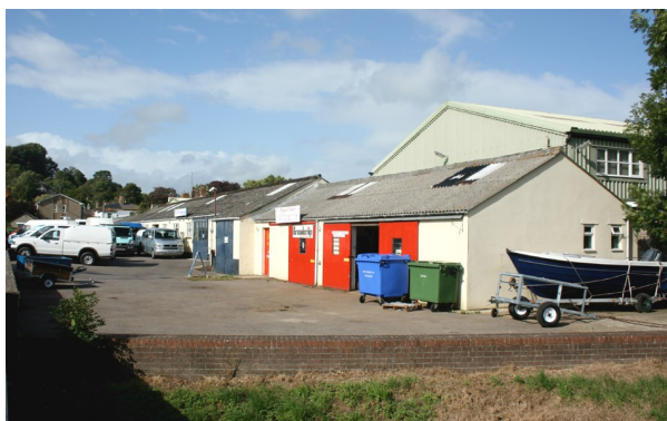
Figure 27: Former Magdalen Works covered rope walk.
