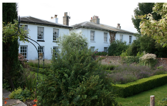
Figure 30: East Road Villas.
