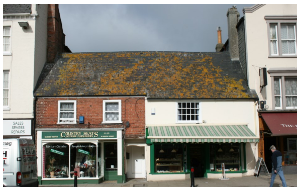
Figure 17: Nos. 16 and 18 South Street.
