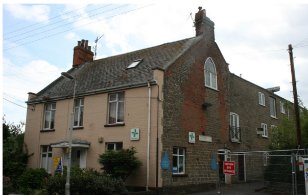
Figure 29: Laurel House, 5 North Allington, formerly Robert Hounsell's house with net loft behind.
