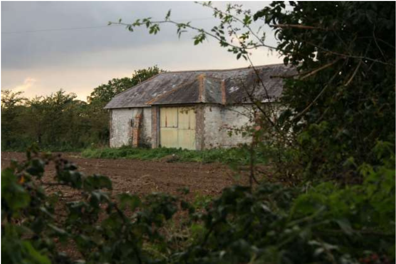
Fig.5.7 Rear of Hurst Dairy Barn (OAA 151015).
