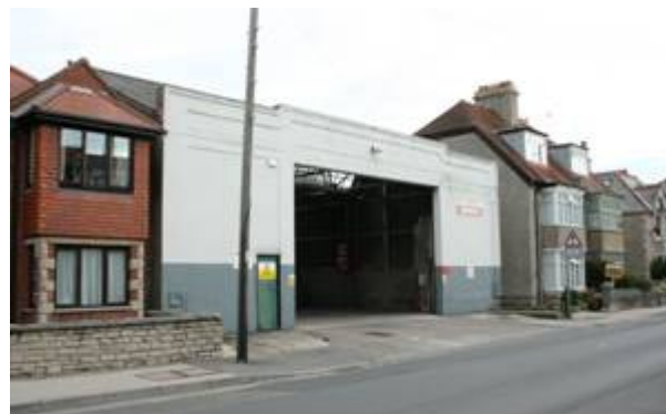
Figure 122: Bus station, King's Road West.
