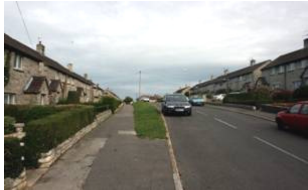
Figure 140: Council housing by Fred Walsh, Priest's Road.
