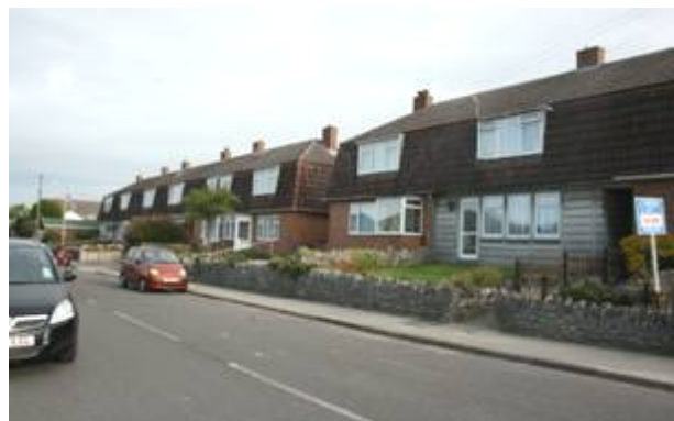
Figure 141: Housing along Priest's Road.
