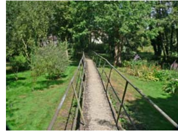
Footpath bridge – Spetisbury Mill
