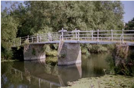
Figure 4: Colber Bridge over the River Stour
