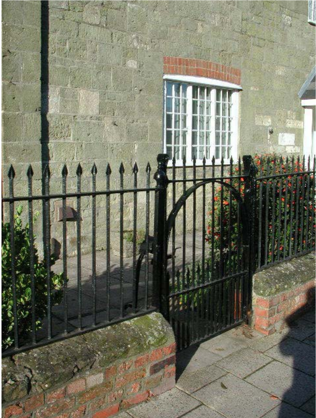
Railings enclosing an existing front yard.
