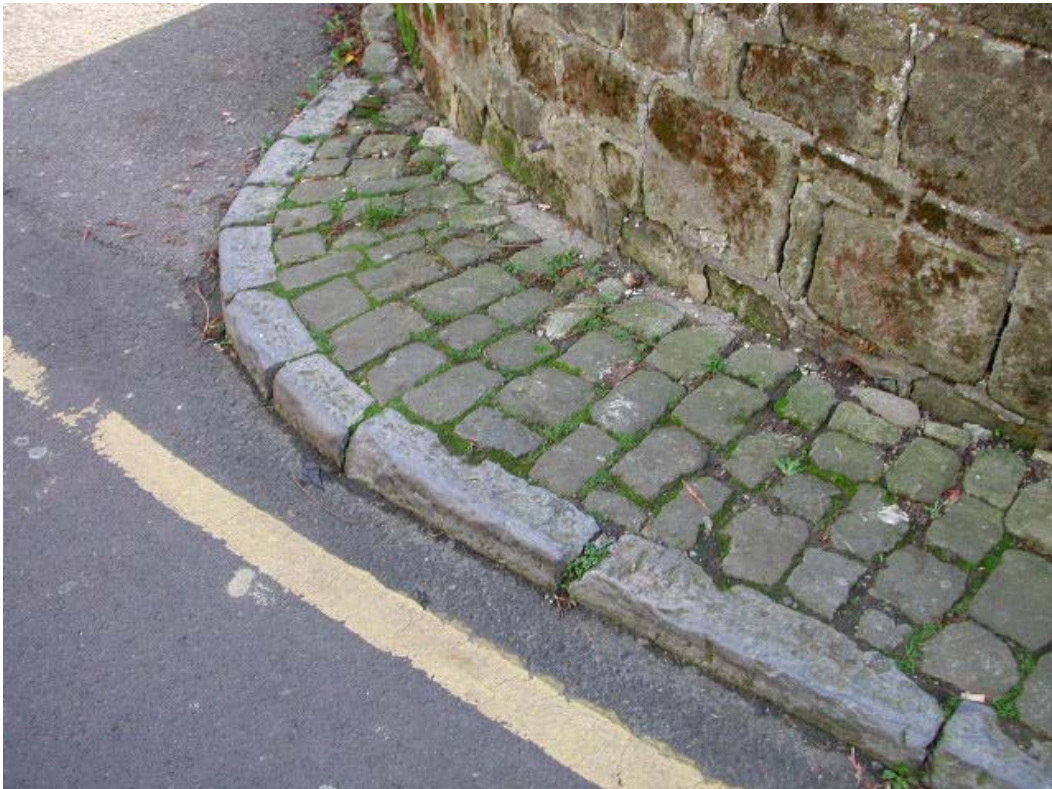
Existing cobbled paving.
