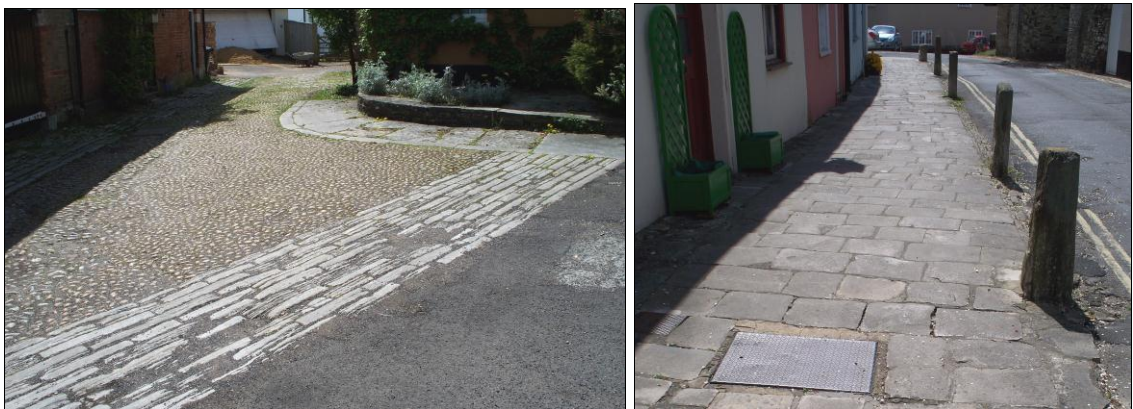
FIG. 12: Historic paving schemes. Left: surfaces adjacent to the old brewery, Pound Lane. Right: paving with stone lined gutter and stone bollards between St John's Hill and Church Green. Both have been damaged by road works.
