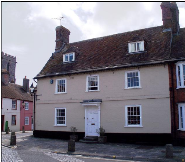
FIG. 14: Three bay format. A three bay configuration expressed at varying scale is common amongst eighteenth century properties. This example in St. John's Hill displays various 'typical' features (e.g. dentil course, stone easing course, hipped dormers, bracketed canopy – multi pane sashes - though the windows appear unusually squat). A stuccoed example is shown in FIG. 8.
