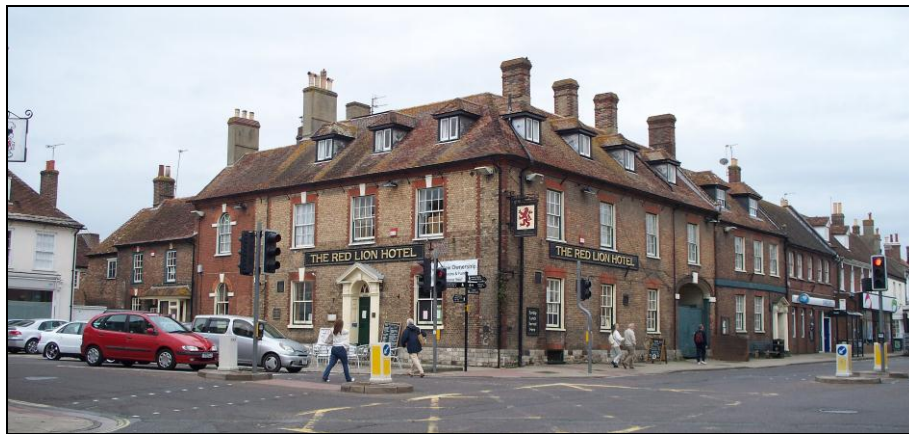
FIG. 9: The Red Lion. A building with strong presence whose bulk in form is balanced by vertical emphasis in detailing and softened by hipping of roofs. The building brings important definition to the corner. The broad gap between this and the town hall was occupied by buildings providing market functions prior to the fire. The location is now dominated by traffic. Note use of buff brick.
