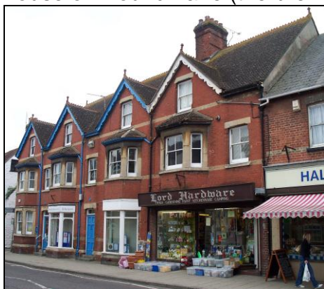
FIG. 6: Late nineteenth century development. A feature most frequent in North Street. The terrace pictured in part replaced the medieval All Hallow's Chapel which stood at the junction with Cow Lane.
