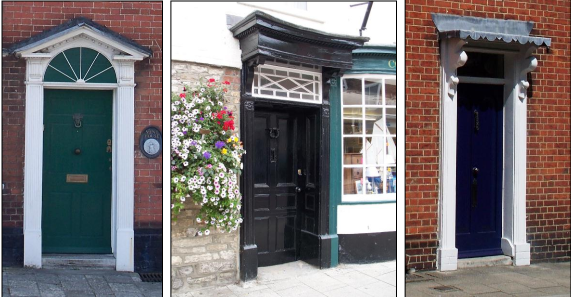
FIG. 17: Door cases. Left: Pilasters with broken pediment and blind fanlight. Centre: bracketed canopy displaying a full entablature with transom light below. Right: simple flat roofed bracketed canopy with transom.
