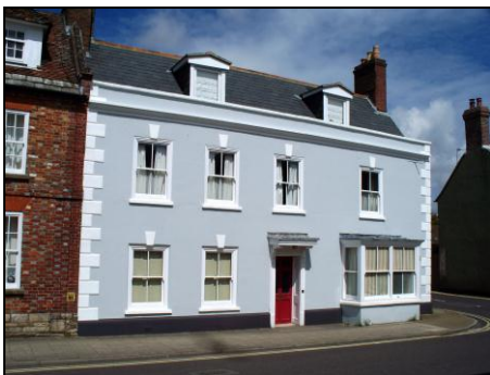
FIG. 15: Stuccoed frontage. A good example of a frontage with parapet, quoins and keystone detailing, though the struck ashlar jointing is no longer very clear. The historic treatment is unlikely to have been pale blue while the bay, dormers, four pane sashes and roof covering all represent later alterations.
