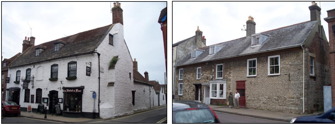
FIG. 4: Buildings of the seventeenth century. Left: 15-17 North Street. Right: 14/14a North Street. It seems likely that the whole of the roof of 15-17 was covered with stone originally, while the slate on 14/14a represents one nineteenth century alteration amongst others (render has clearly been removed from the frontage).
