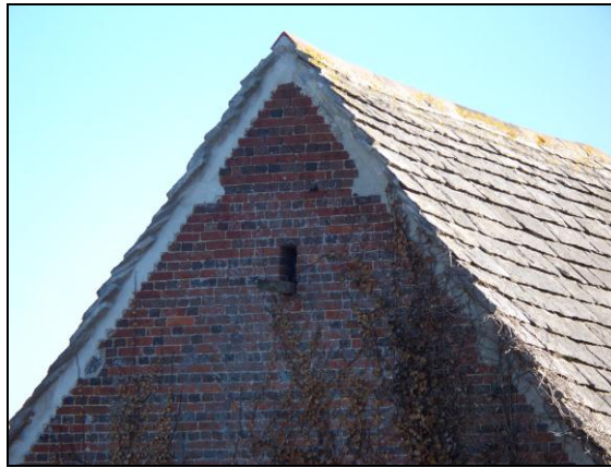
FIG. 12: Barn owl nesting slot and perch. Seen in the end gable of the barn opposite Manor Farm Cottage.
