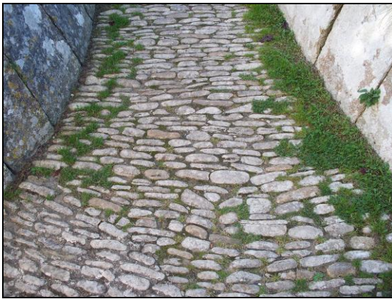
FIG. 6: Churchyard paving. The stone slab revetment of the banks either side is also interesting.
