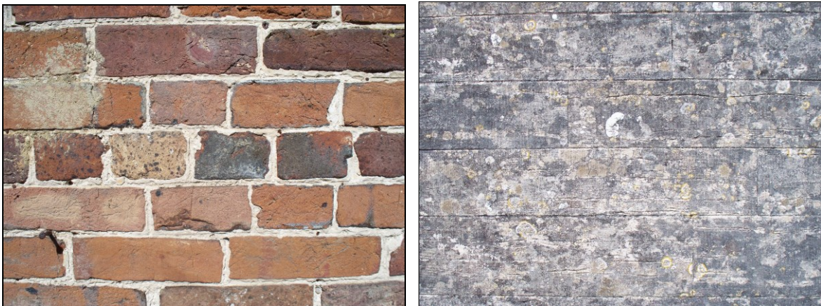
FIG. 13: Typical building materials. Left: brick. Note the variations in the tone of red reflecting variable conditions during firing. Right: finely jointed blocks of Portland stone (termed 'ashlar').
