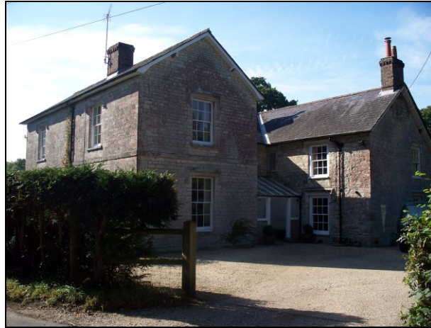
FIG. 16: Manor Farm. The original house is the range to the right, and probably dates to the early nineteenth century. The range to the left and centre is a large extension probably added later that century. The quality of construction and retention of many original windows is notable. Reflecting the different dates of the two parts of the property, the windows on the older range have exposed sash boxes, whilst those on the later range are recessed.
