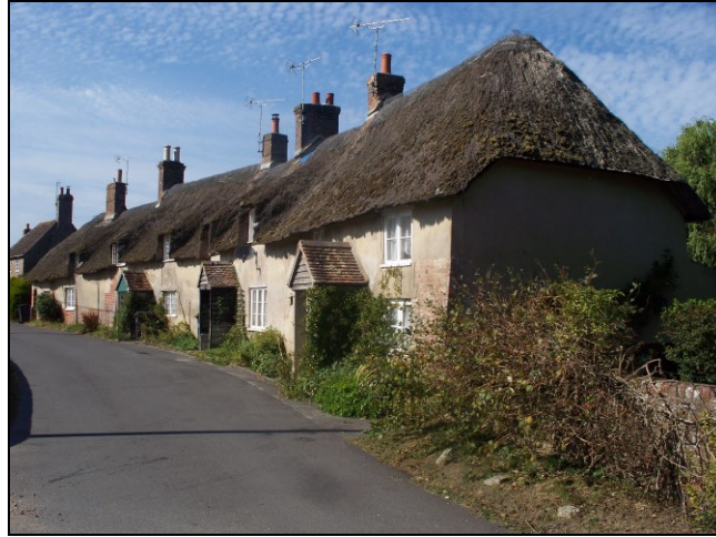
FIG. 14: Thatched roofs of Nos. 2-5 The Street.
