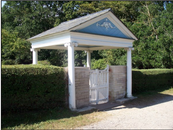
FIG. 4: Classically styled gate to the new cemetery. Originally constructed c.1800 as entrance to the kitchen garden, and moved here c.1950. The modern brick walls either side incorporate panels taken from the obelisk on Fir Hill.
