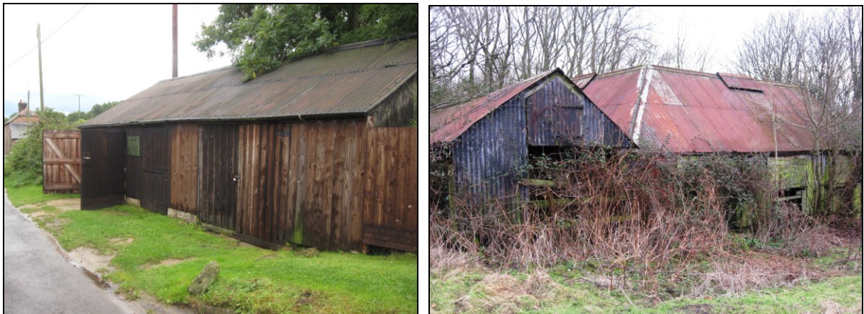
FIG. 28: Timber boarding and corrugated iron. Left: shed at 47 West Morden featuring the distinctive use of vertical timber boarding. Corrugated iron covers the roof. The latter is frequently seen around the conservation area as a partial or full cladding as in the semi-derelict structure located at Shrubets (right).
