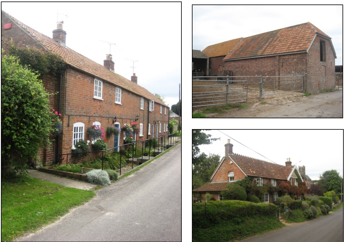
FIG. 31: Double Roman tiles. As seen on the roofs of Nos. 64-67 Higher Street (left), a building at Hill Farm (top right) and the Old Post Office Higher Street (bottom right).
