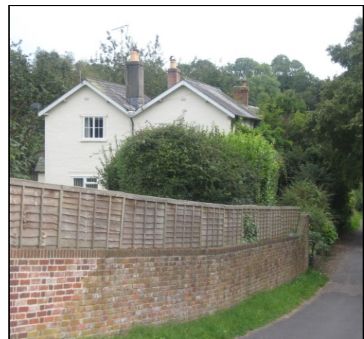
FIG. 29: Varied roof forms. Top left: Pitched roof with rear catslide at No. 165. Top right: half hipped thatch roof of No. 76 Higher Street. The slate roof of No. 74 adjacent appears to have replaced a roof similar to that at No. 76. Right: 'M' shaped roof at No. 69 Higher Street.
