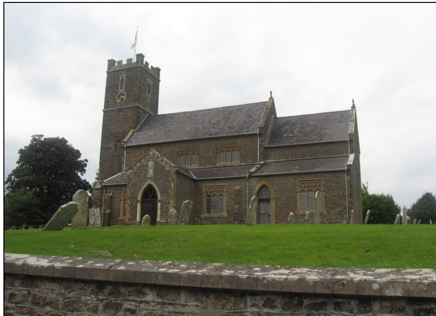
FIG. 1: St. Mary's Church, Higher Street. A picturesque and well positioned building, the church is of particular interest as for being almost entirely constructed from heathstone. Little remains of the medieval church it replaced.
