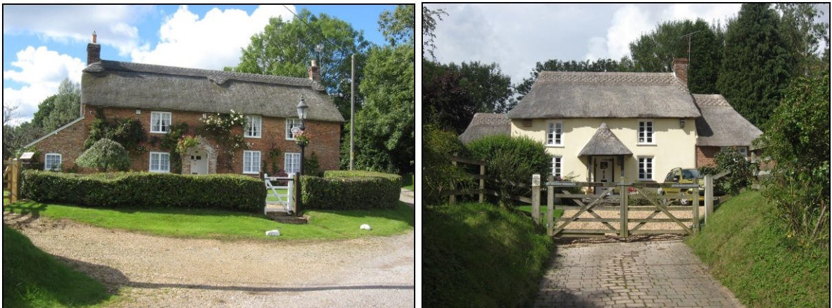
FIG. 11: Thatched buildings at Whitefield. No 153 and Whitefield Farmhouse. Note the contrast in ridge styles – a flush ridge is the local traditional finish.
