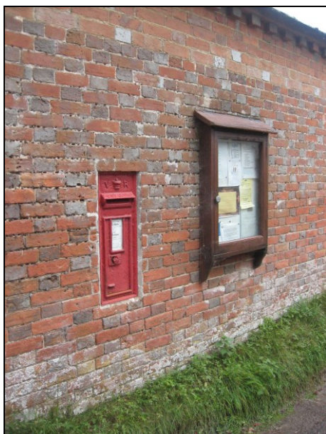
FIG. 32: Street furniture. Left: Pillar box in West Morden. The Victorian box is fitted into the wall of an agricultural building at King's Corner Farm. Note the chequered Flemish bond brickwork using red stretchers and blue headers. Right: Finger post at the Cock and Bottle. Two fingers have clearly been replaced, but it retains its original roundel which records the location. The appearance of the post is spoiled by the speed sign attached below. Surprisingly the speed limit here is 60 mph.
