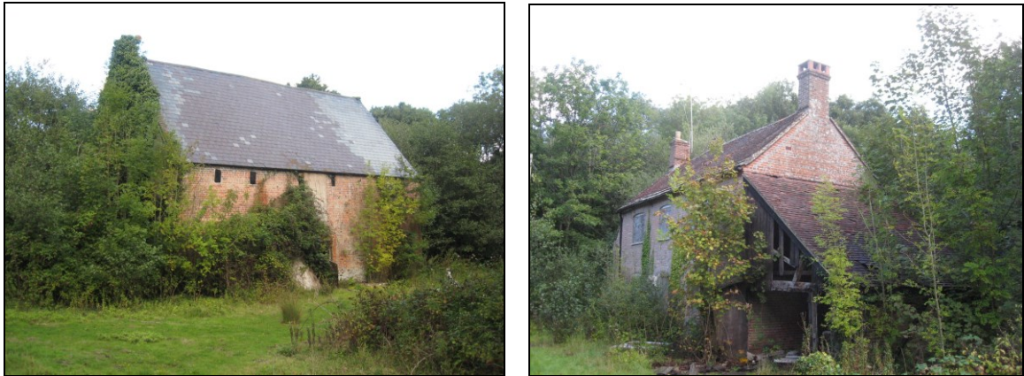
FIG. 14: Morden Mill and Farmhouse. Derelict listed buildings, albeit the farmhouse was inhabited until recently. Note the attached timber framed and clad outbuilding – a common feature of Morden Estate properties around the conservation area. Maps reproduced with the permission of the National Library of Scotland.
