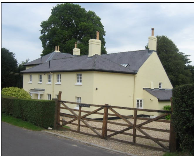
FIG. 30: The Old Vicarage, Higher Street. The roof of this building has recently been re-covered with Welsh slate. The original part of the property is to the rear and can be identified by the steeply pitched roof with catslide – similar to others within the conservation area. Clay tiles are likely to have covered the oldest part of the building originally, though slate would have suited the lower pitches used when enlarged during the nineteenth century.
