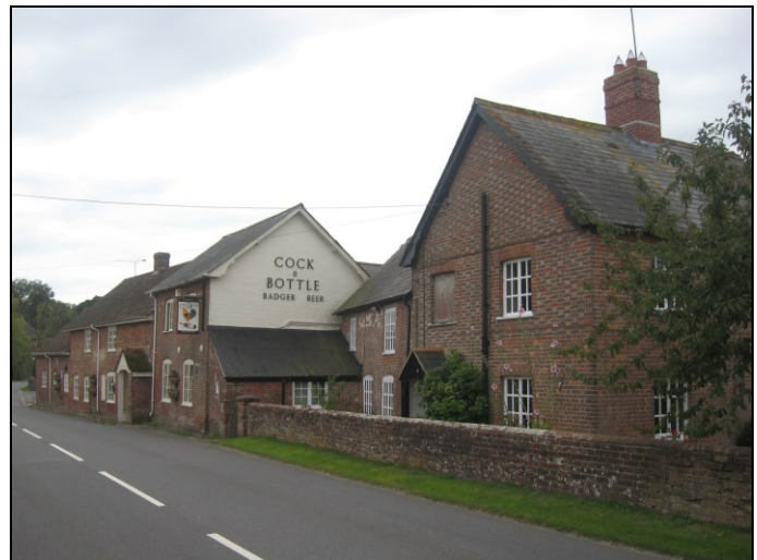
FIG. 17: East Morden building frontage. This is one of only two continuously developed frontages in the conservation area. Variation in building form, orientation and height here provides visual interest.
