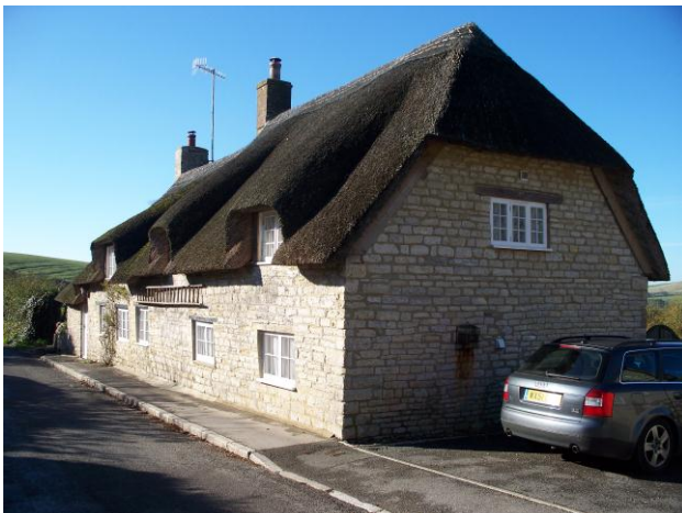
FIG. 2: No. 20. The cottage has its origins in the seventeenth century, albeit altered and extended later. The pronounced lines of the two dormers to the right are one indication that the building has been rethatched. The old village 'fire ladder' hangs on the front wall.
