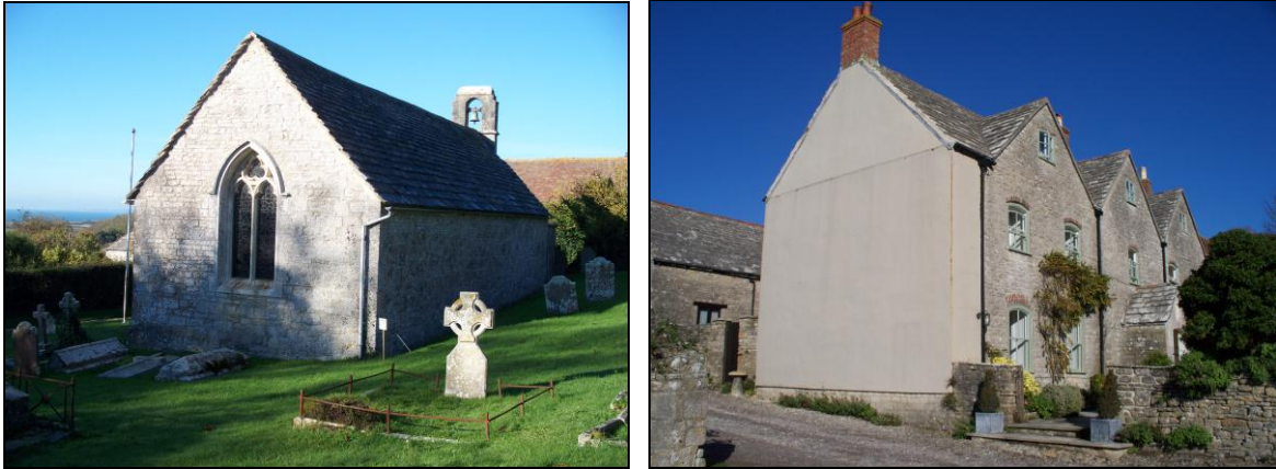
FIG. 10: Buildings at the top of the village. Construction of both walls and roofs in Purbeck stone characterises development here, in contrast to the pattern seen in the village below.
