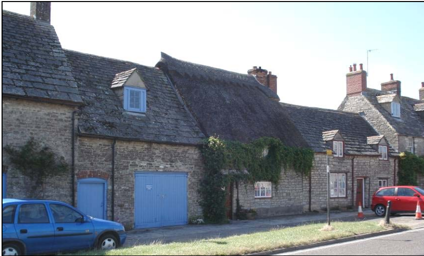
FIG. 5: Variety. Variation in height, roof covering and the arrangement of openings is seen along the middle section of East Street. Note the unenclosed forecourts.
