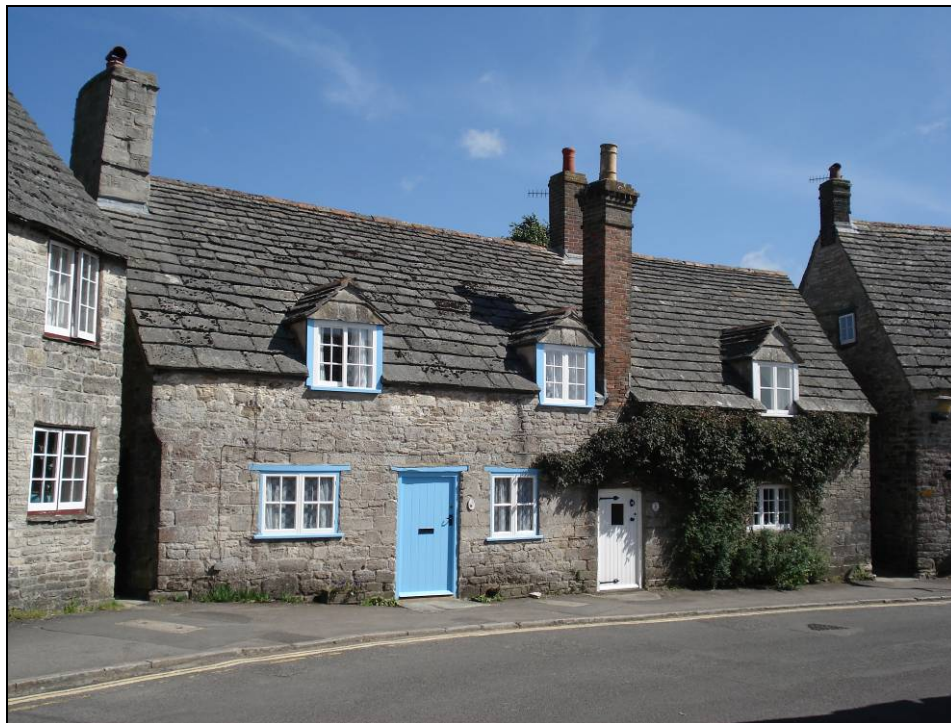
FIG. 10: The vernacular. 17/19 West Street, formerly a single house dating to at least the seventeenth century – and thus possibly utilising stone from the castle – displays many of the key features. Note the chimneys, one of ashlar, two of brick, that on the front elevation an odd eighteenth century addition. Windows are relatively regular though include a mix of casement and horizontal sliding sash, while dormers sit below the eaves.
