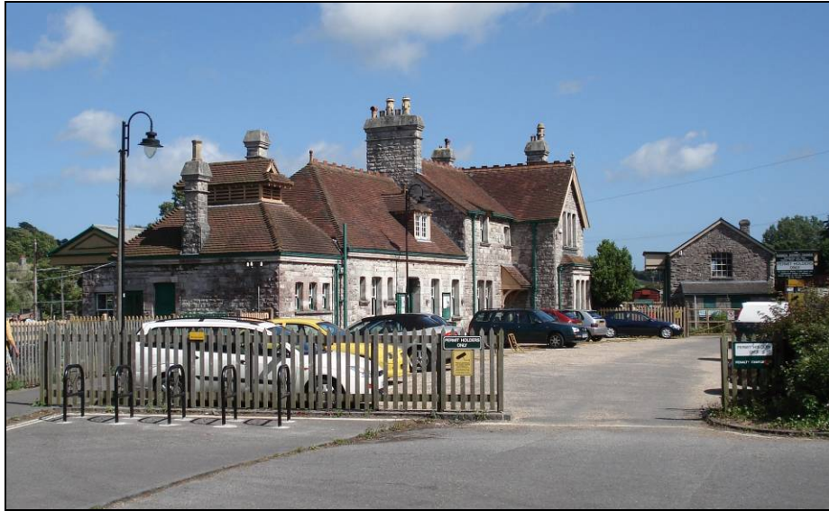
FIG. 3: Corfe Castle Railway Station and goods shed. A good example of a historic village station. The reproduction arc lamps are perhaps incongruous.
