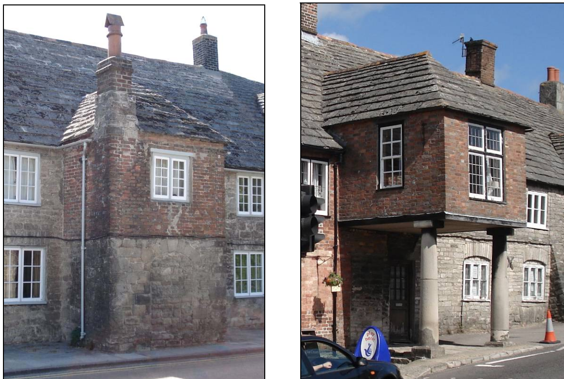
FIG. 9: Two storey porches. Left: A fully enclosed porch at 64 East Street. These are otherwise seen at the Town House and Morton's House. Right: two storey porch with open ground floor, also seen at the Greyhound.
