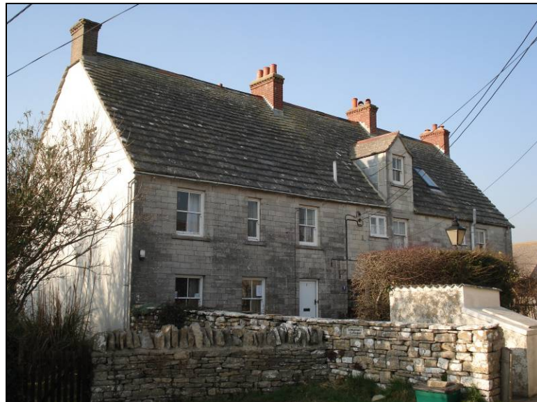
FIG. 8: Late Victorian development. With form and appearance of more standardised ‘urban’ character this building nonetheless employs local materials in construction including in this instance Swanage brick for chimney stacks. Note the awkward looking dormer.
