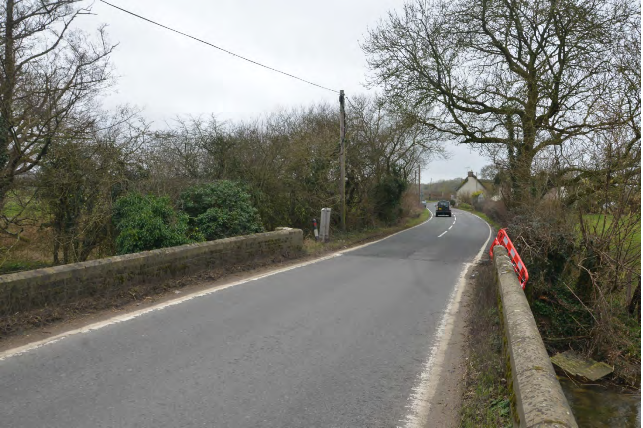
Plate 25: View of Hurst (South) Bridge
