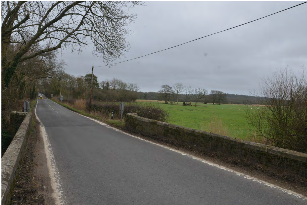
Plate 24: View of Hurst (South) Bridge
