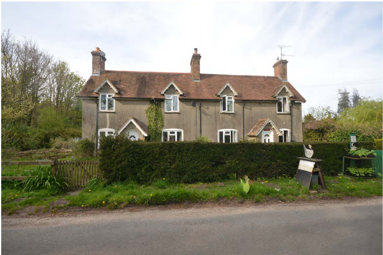
Plate 9: View of Daisy Cottage, Station Rd
