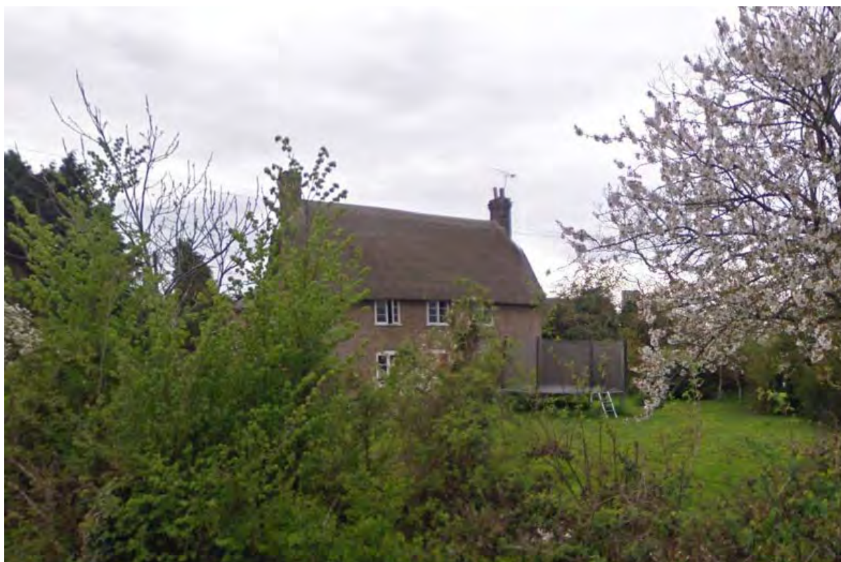
Plate 44: View of Hurst Dairy House / Dairy Cottage (Google Street View)
