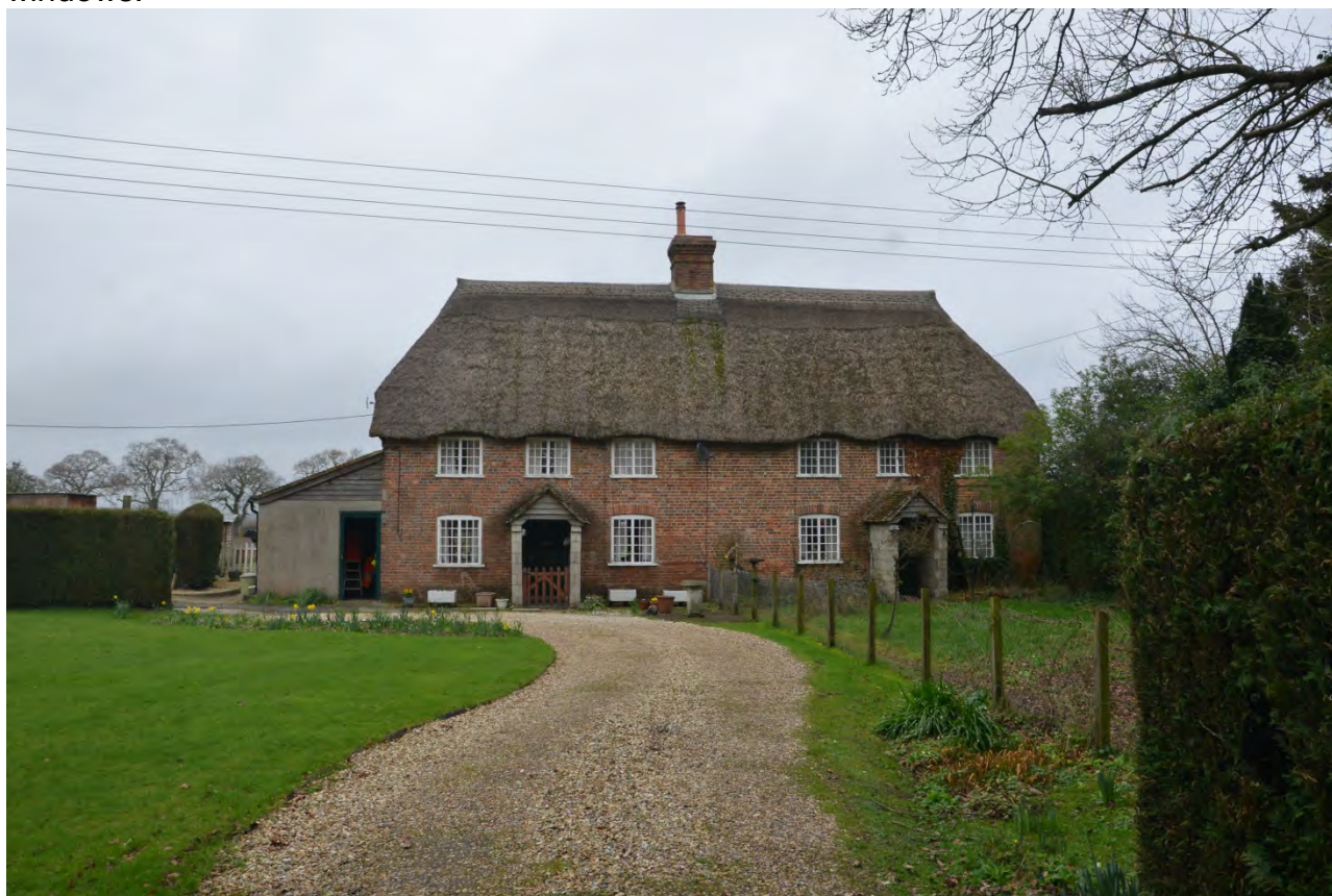
Plate 6: View of Manor Farm Cottages Station Rd
