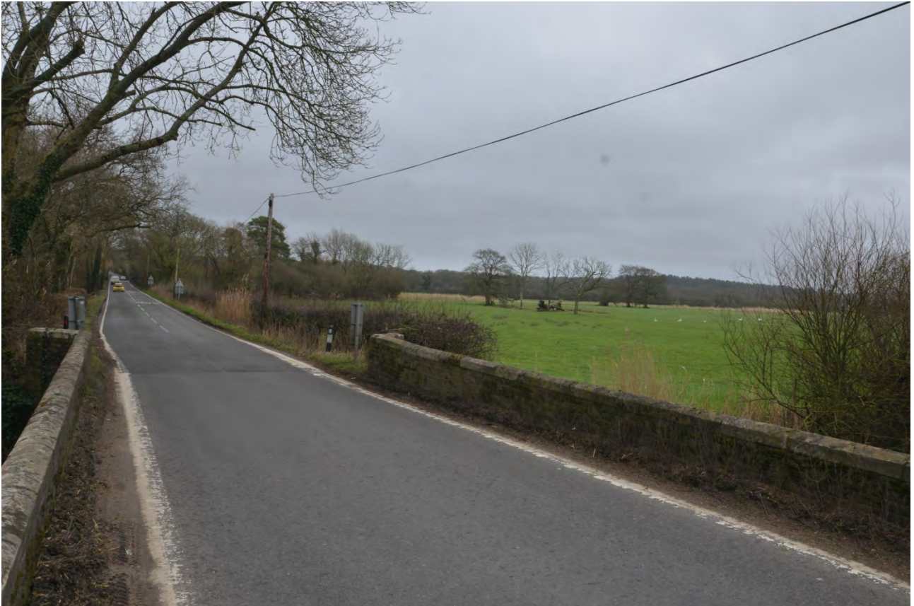
Plate 39: View of Hurst (South) Bridge
