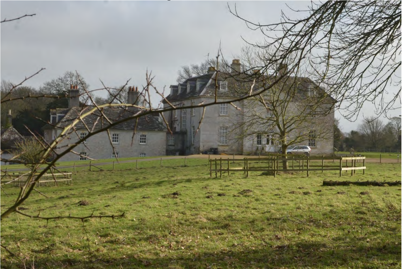
Plate 13: View of Moreton House Hurst Rd
