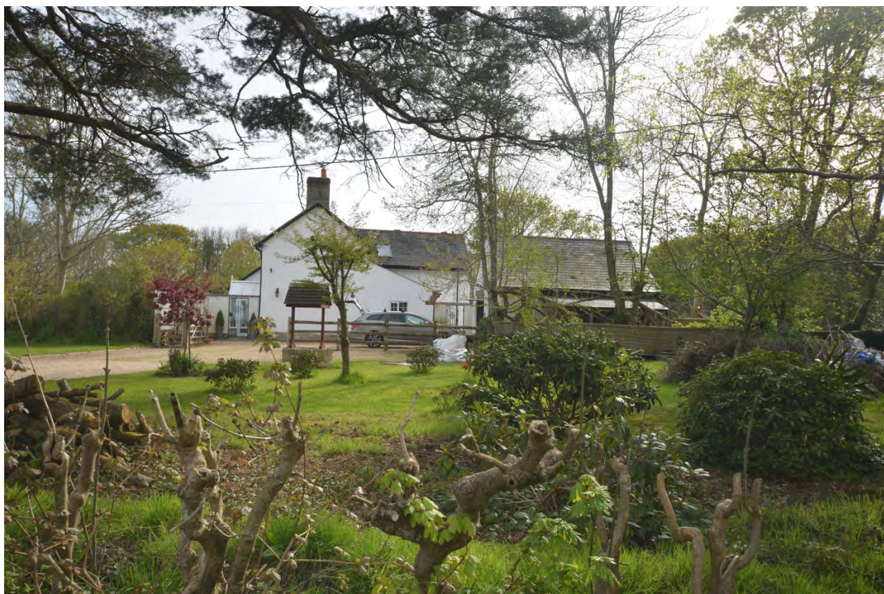
Plate 32: View of Fir Tree Cottage The Common
