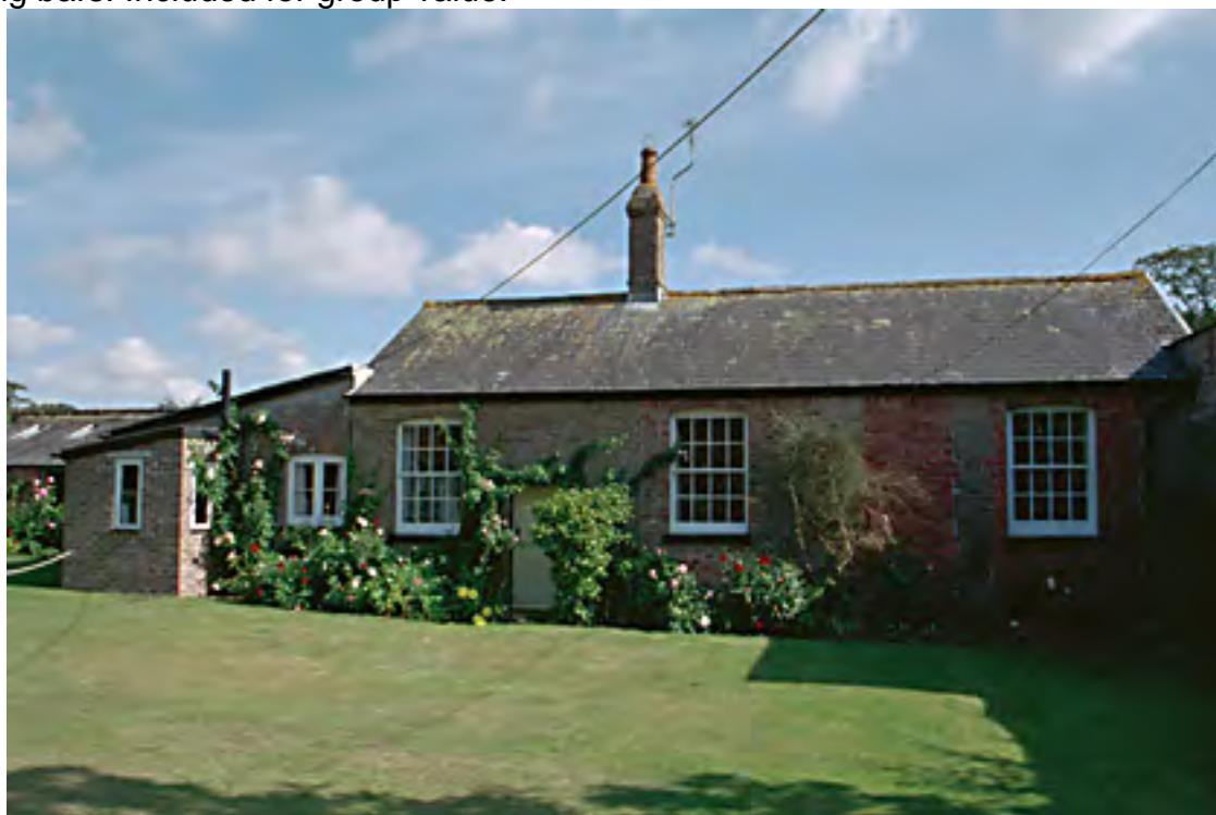
Plate 16: View of Gardeners Cottage at Glebe House Hurst Rd (Images of England)
