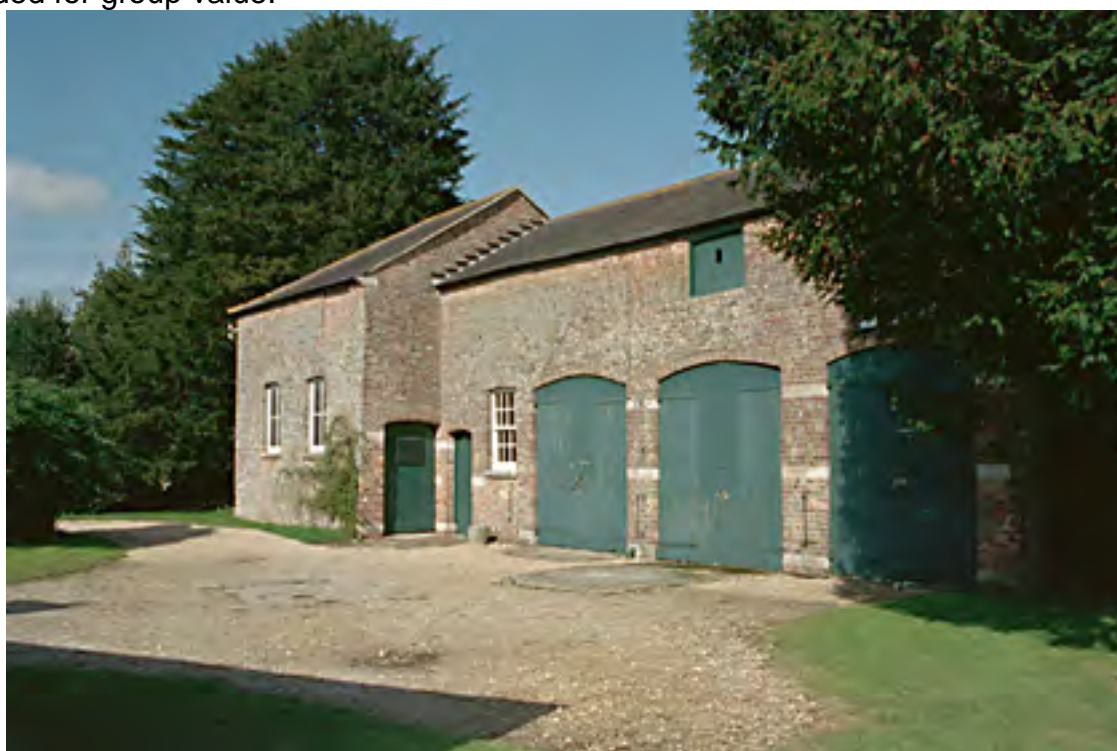
Plate 17: View of Stables & Coach house at Glebe House Hurst Rd
