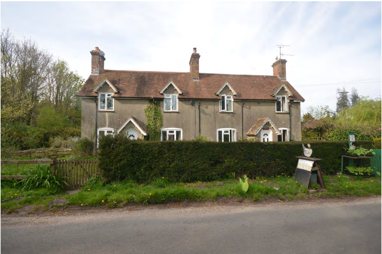
Plate 33: View of Daisy Cottage, Station Rd
