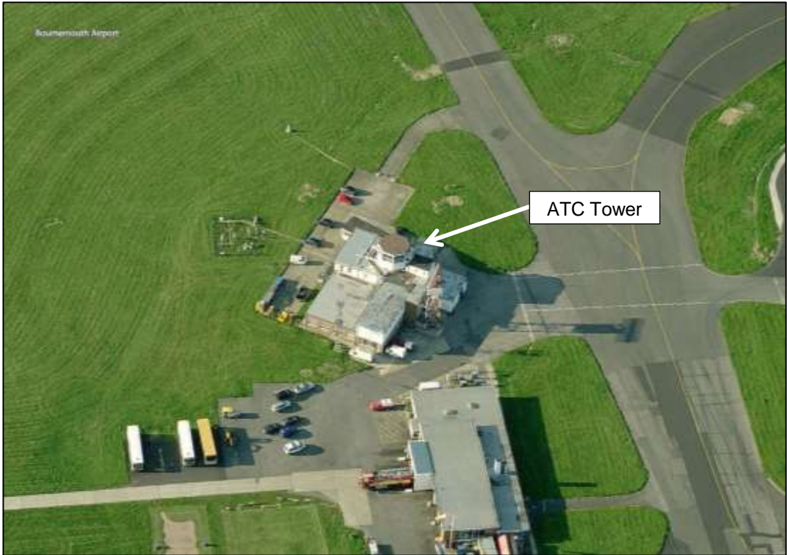
Figure 8 ATC Tower location- zoomed
